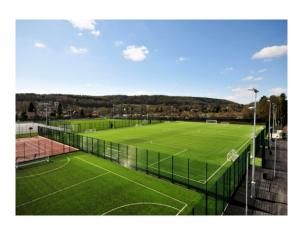
White Horse Contractors (Northern) Ltd were appointed to construct a  $106m \times 70m$  and a  $37m \times 21m$  sand & rubber filled artificial turf pitches to be marked out for football and 5 a side and hockey, complete with fencing and floodlights. The ATPs were part of the pitch development constructed by White Horse that included macadam MUGAs and a natural grass pitch.
