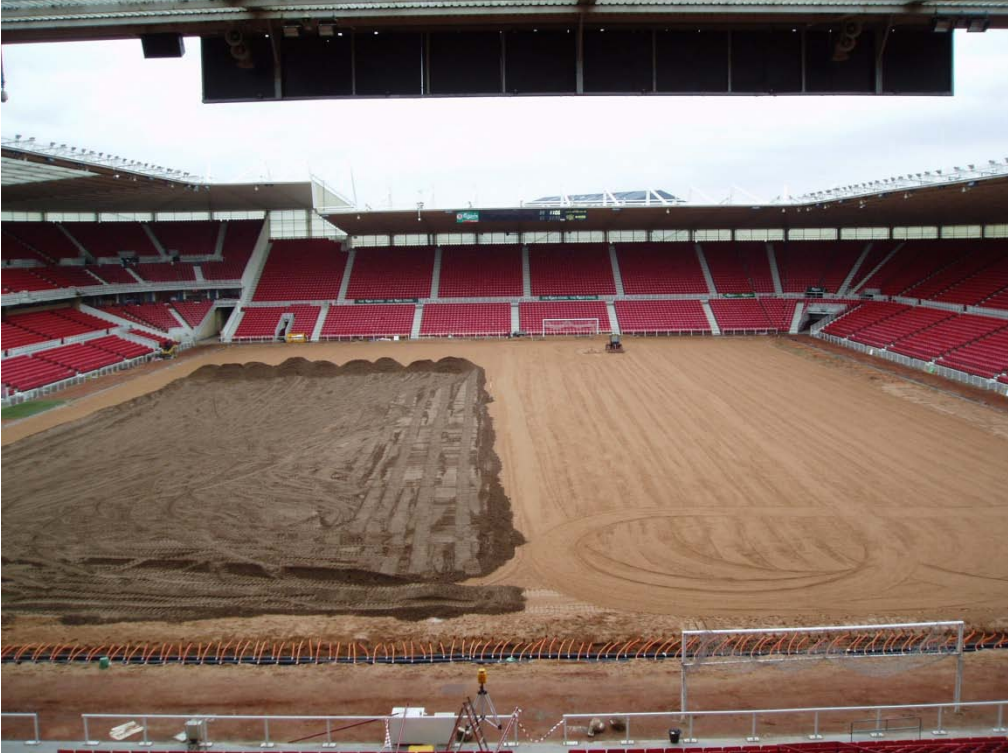
Top root zone layer placement
