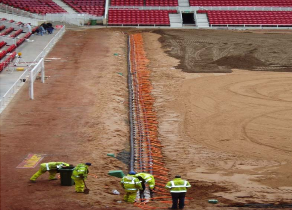
Under soil heating pipe installation
