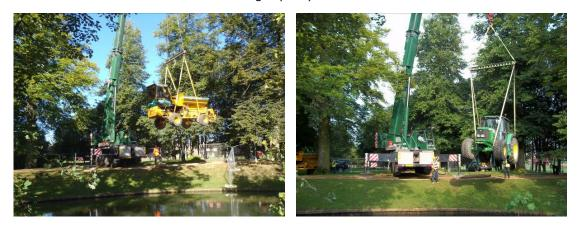
In our workshops, the firm had to strip down our plant and equipment in order for the crane to manoeuvre their machinery to the sports field to begin work. Over the course of 2 days up to 12 loads of equipment and 300 tonnes of gravel were delivered to a tight schedule by Smiths of Bletchington. Each lift had to be controlled in order that river traffic could continue.
