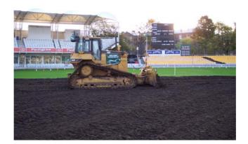
By using its own Mastenbroek 10/12D trenching equipment, White Horse Contractors was able to carry out the main drainage works, installing more than 3.6km of lateral drains and 294m of ring drains. These pipe trenches were later backfilled using CT12 crawler trucks. Due to the speed with which the machines were able to handle the scale of the site the final pieces of turf were laid on schedule, ensuring the outfield would be ready for use soon after.
